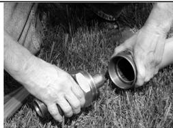
2. Disassemble compression nut, retainer, gasket, lock ring and stiffener from body. Read markings on pipe, stiffener and gasket. Pipe must read D2513. Pipe, gasket and stiffener must all be 1-1/2" IPS. Make sure SDR 11 (wall thickness) marked on stiffener matches SDR of pipe.
