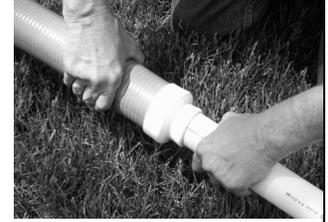
5. Slide compression nut, then retainer, then gasket, then lock ring onto pipe.
