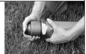
10. We recommend that red line on casing be above ground after final grade. (See Photo at left.) Test assembly per local requirements.
