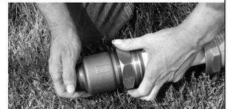
8. Use two 24" (or larger) pipe wrenches to tighten compression joint by holding body stationary with one wrench and tightening compression nut with other. Apply at least 65 pounds of force to ends of 24" wrenches when tightening compression nut.
